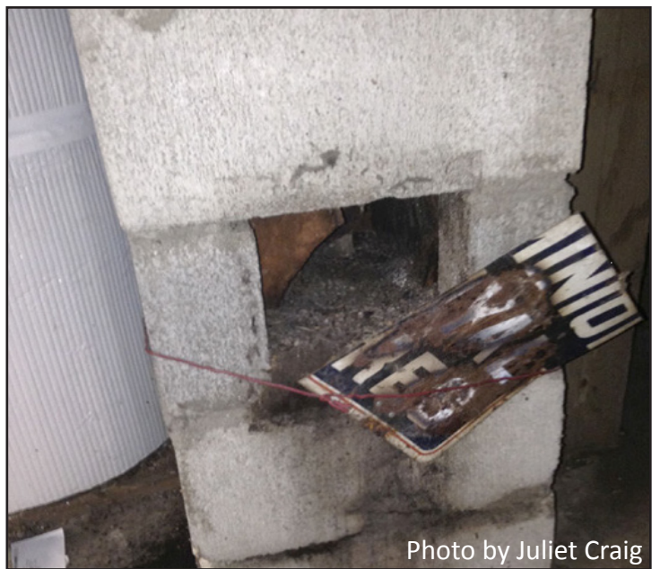
Figure 33. A chute sealed at the bottom instead of the top.
